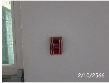
Fire Alarm Manual Station
