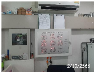
Graphic Annunciator Fire Alarm System
